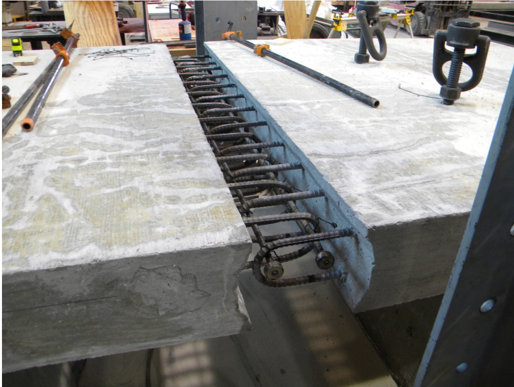
Figure 3.13: View of completed joint prior to pour
