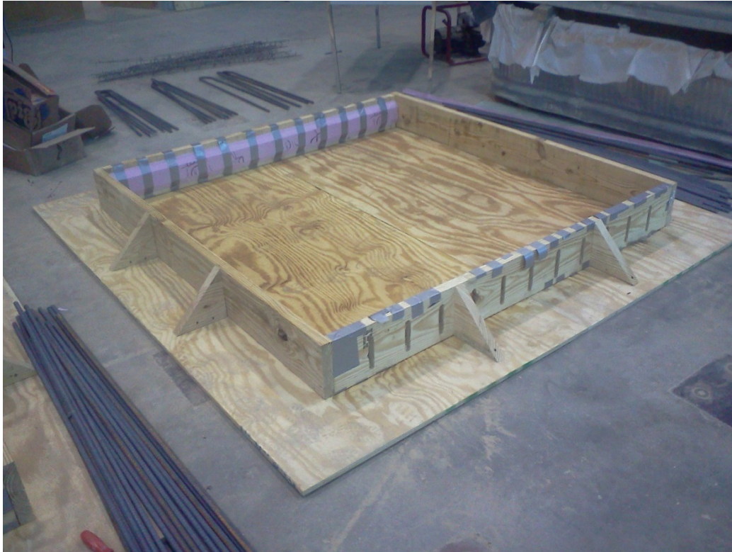
Figure 3.5: Specimen formwork with foam board for shear key
