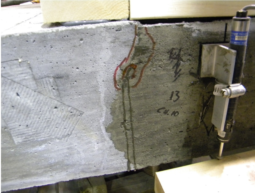
Figure 3.25: Leaking at end of joint
