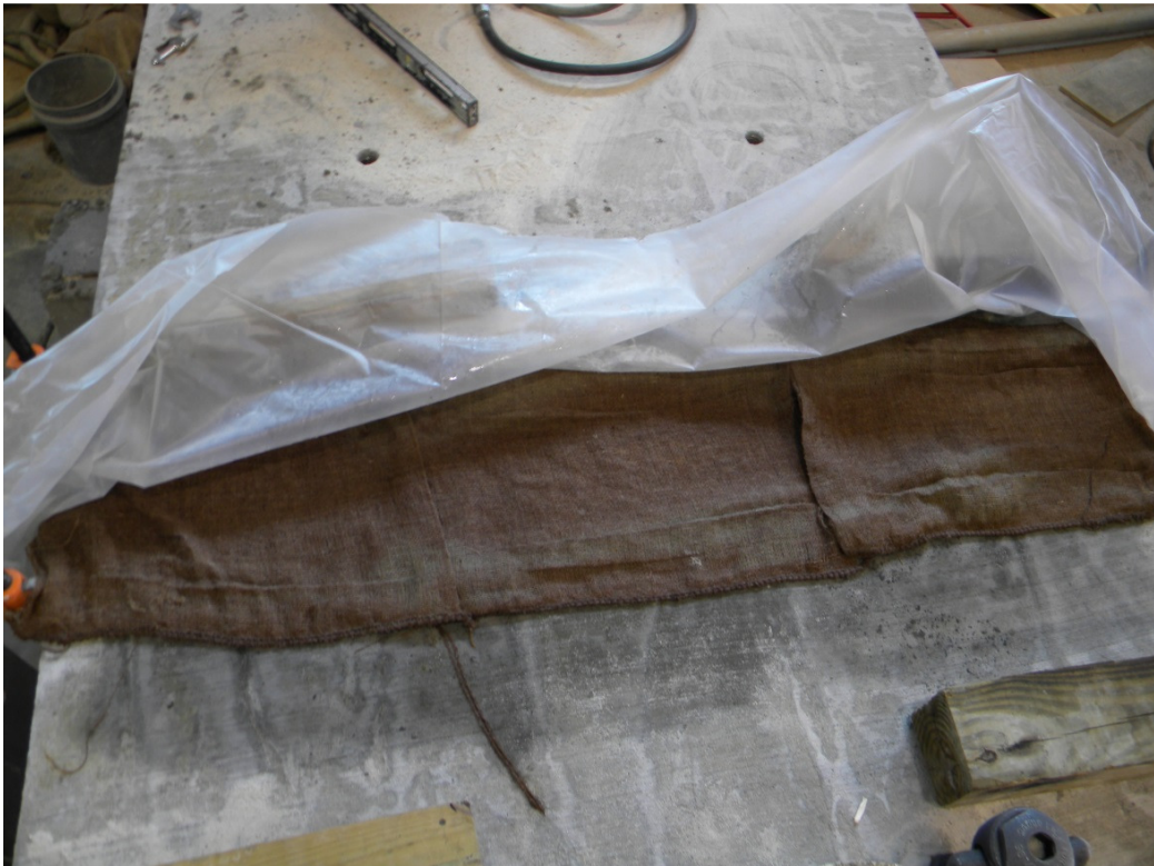
Figure 3.16: Burlap and plastic used for curing joint
